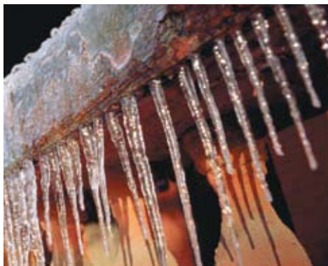
Gutter without cable and Ice & snow detector
